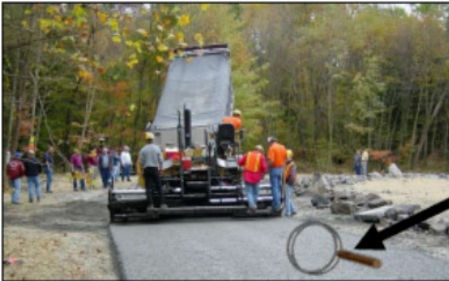
Figure 1: Placement of DSA through a paver.
