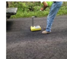
Figure 4 - Compaction Testing with Nuclear Density Gauge
