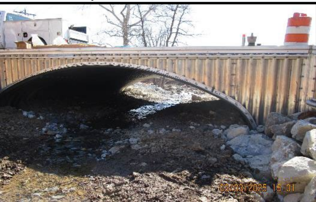
Just completed to standard in Adams
