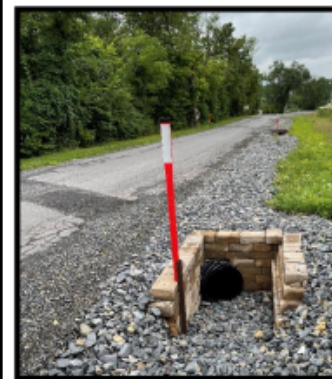
Cross pipes are commonly used in DGLVR projects to direct water away from the road and nearby streams.
