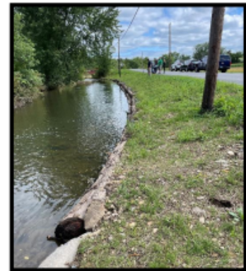
Public roads that drain to streams or otherwise impact water quality are likely eligible for DGLVR funding.
