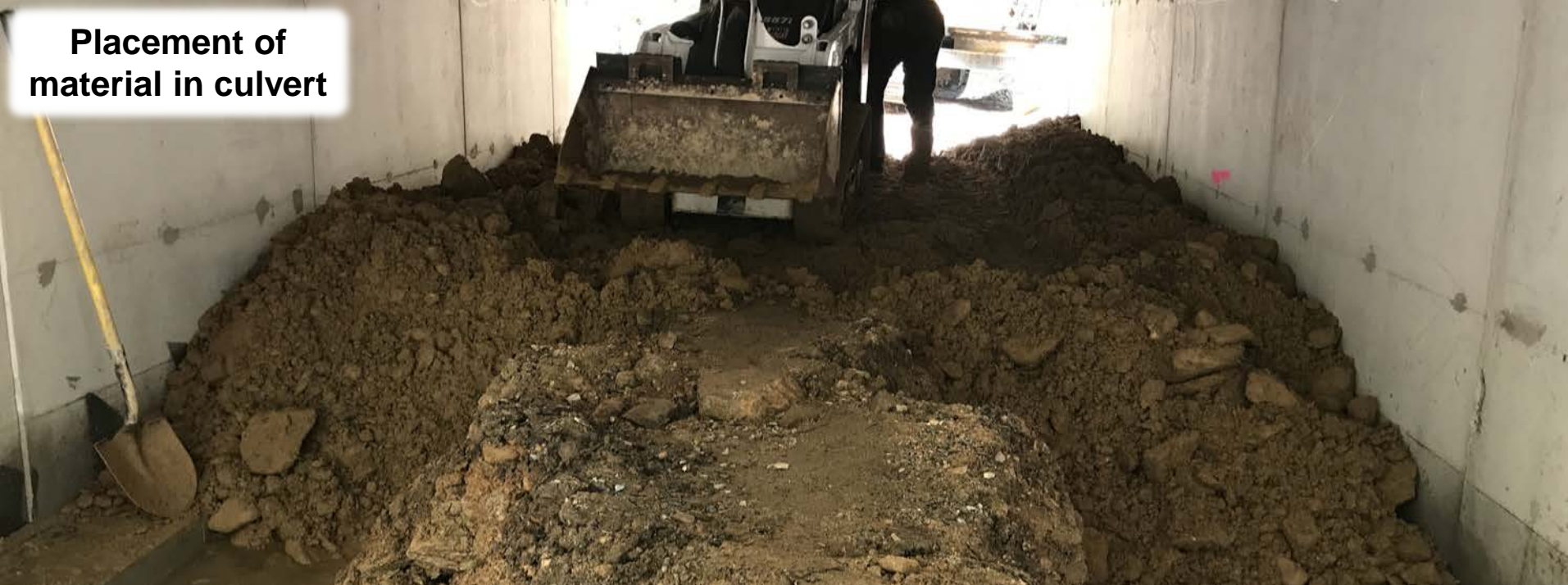
Washing of fine into culvert fill material
