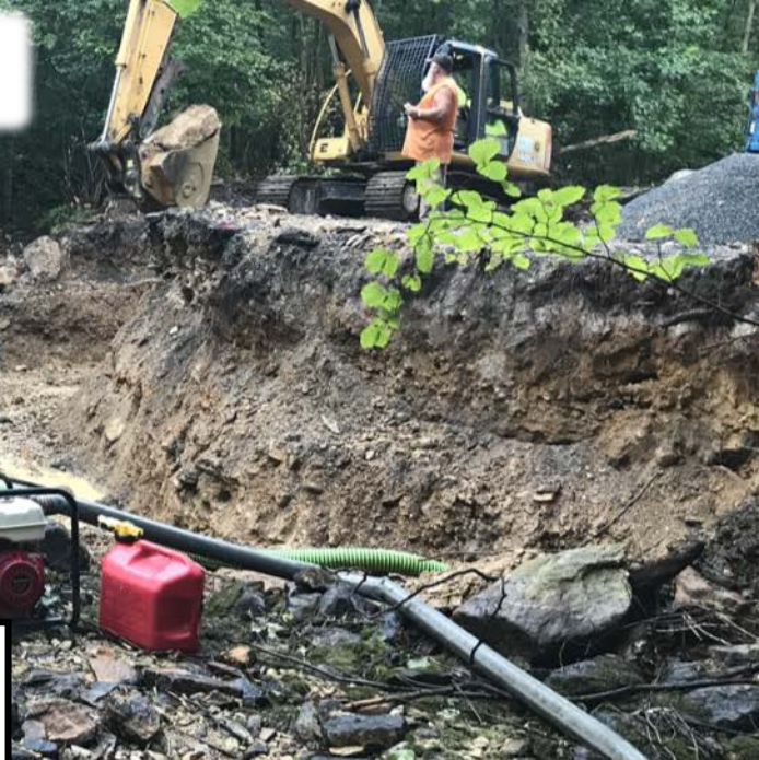
Excavation for new culvert
