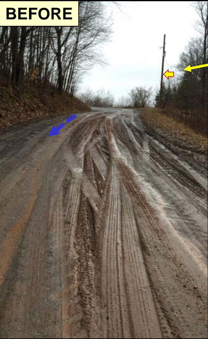
After base addition, before surface
