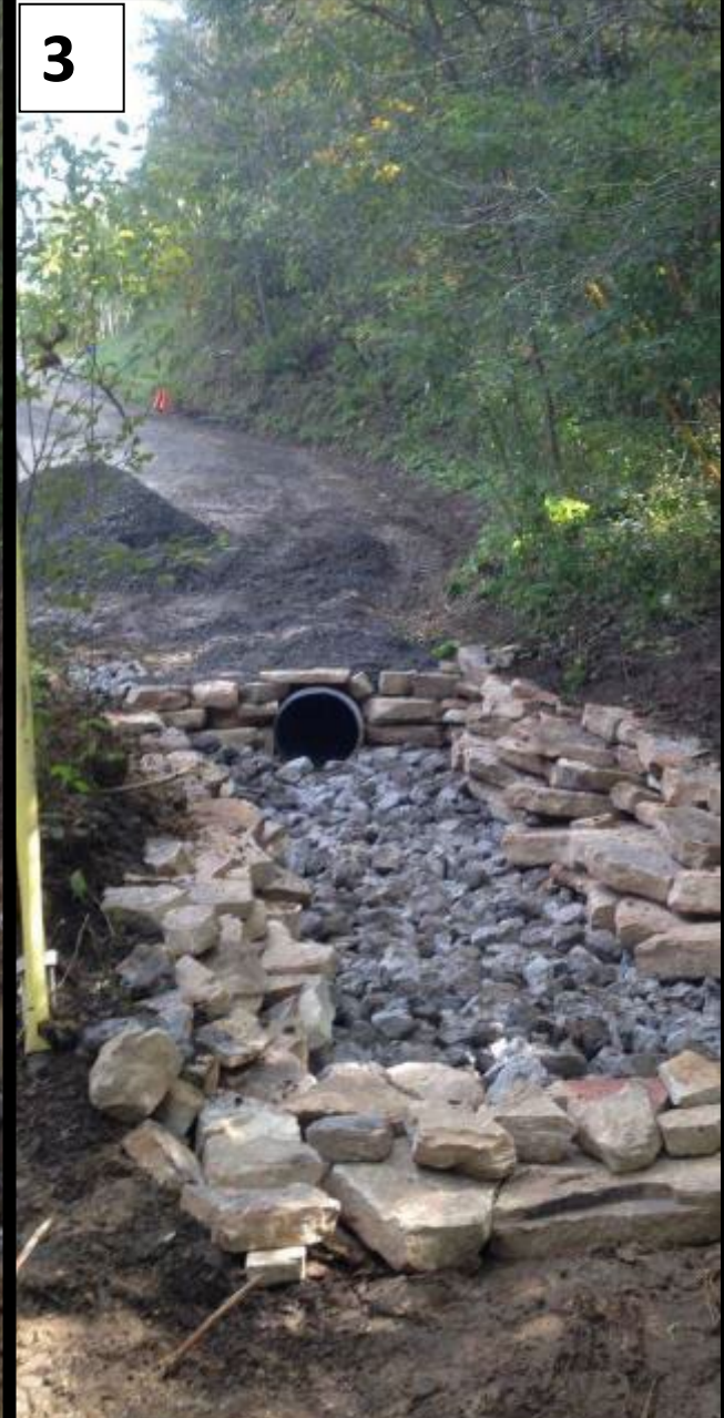
3' Deep, filled w/ R4 and edged with pallet stone.
