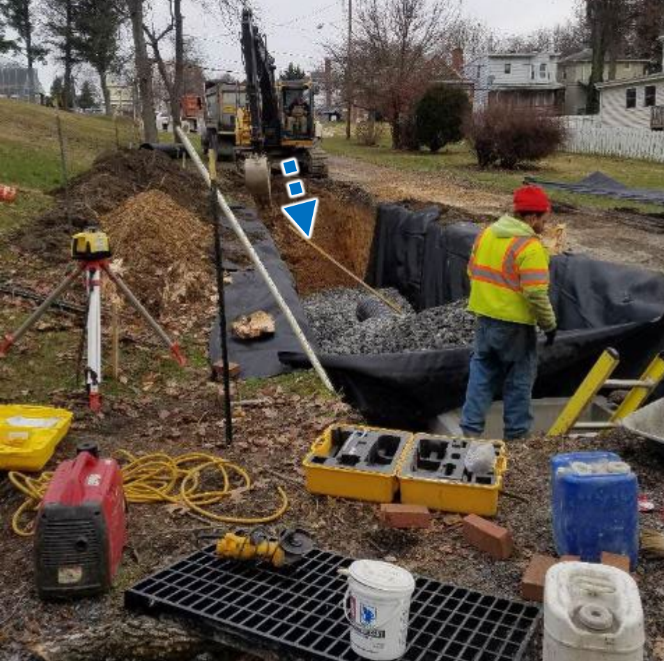
Dauphin, 31 st St 6/7 • Installed drop inlets to “cascading” subsurface infiltration structures
