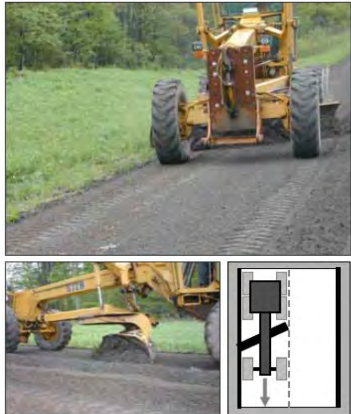
Figure 25. Large aggregate that has accumulated on the shoulder is pulled to the center of the road and mixed with fine aggregate particles as it rides up the blade. The blended aggregate is deposited in a wind-row in the center of the road. Note the high moisture content of the graded material.
