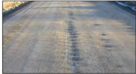
Figure 20. Potholes.
