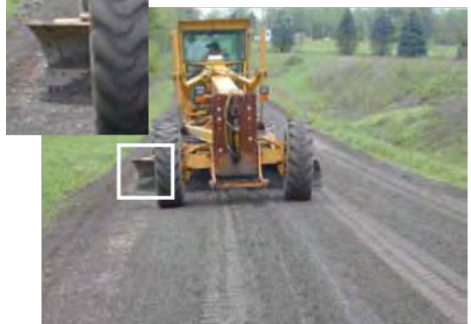
Figure 31. Grader grooming the road. Notice the grader blade is not carrying a lot of material.
