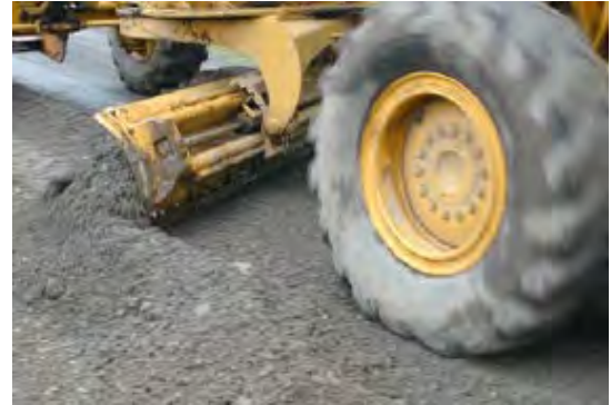
Figure 24: Wet material rolling off blade.
