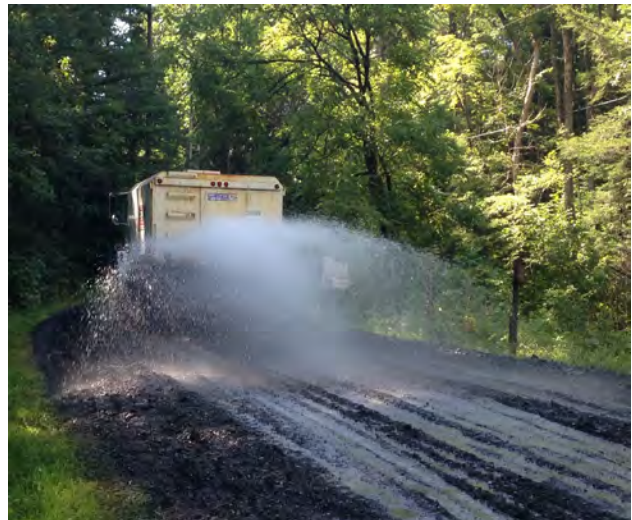
Figure 27. Adding water to a dry road surface.
