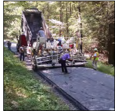
Paver placement of DSA.
