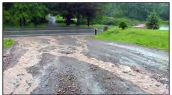
Figure 19. Water in wheel tracks.
