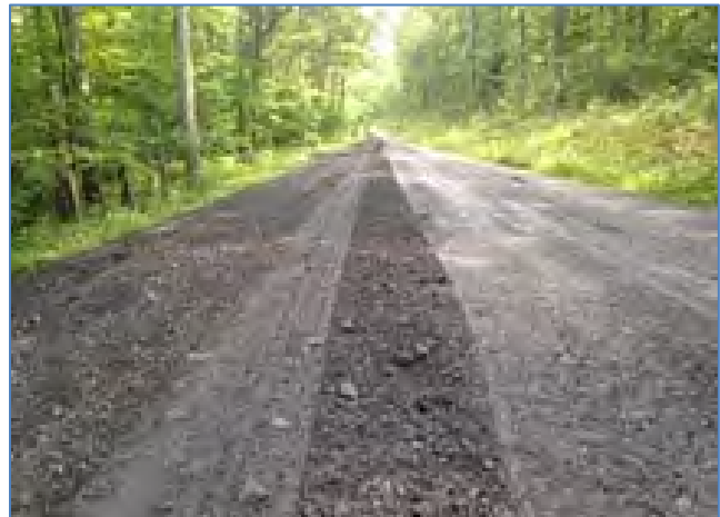
Figure 32. Before & after first pass of 10-ton roller.
