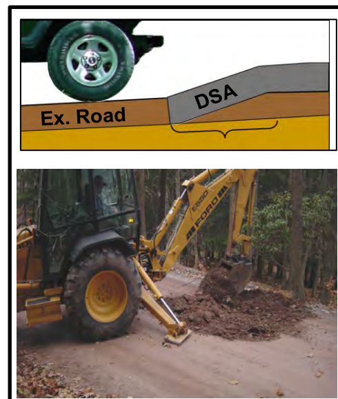
Figure 11. Paving Notch cut across road to support end of placement.
