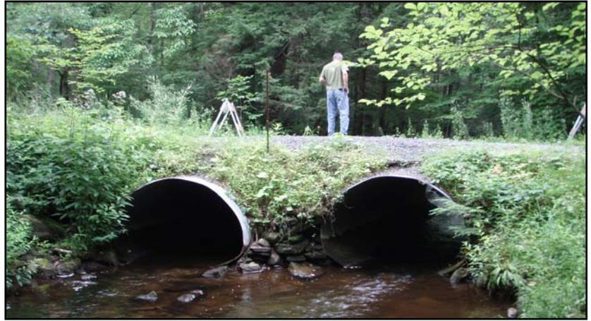
Photo 3. One of the stream crossings is pictured here. Both crossings have identical sized double pipes. Water flowing over this pipe in high flows has eroded the unprotected crossing, which is why you see construction barriers on the road.
