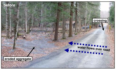
Photo 1. When the undersized stream pipes reache capacity, water flows over the road at this point. Large quantities of aggregate are routinely washed into the floodplain and stream.
