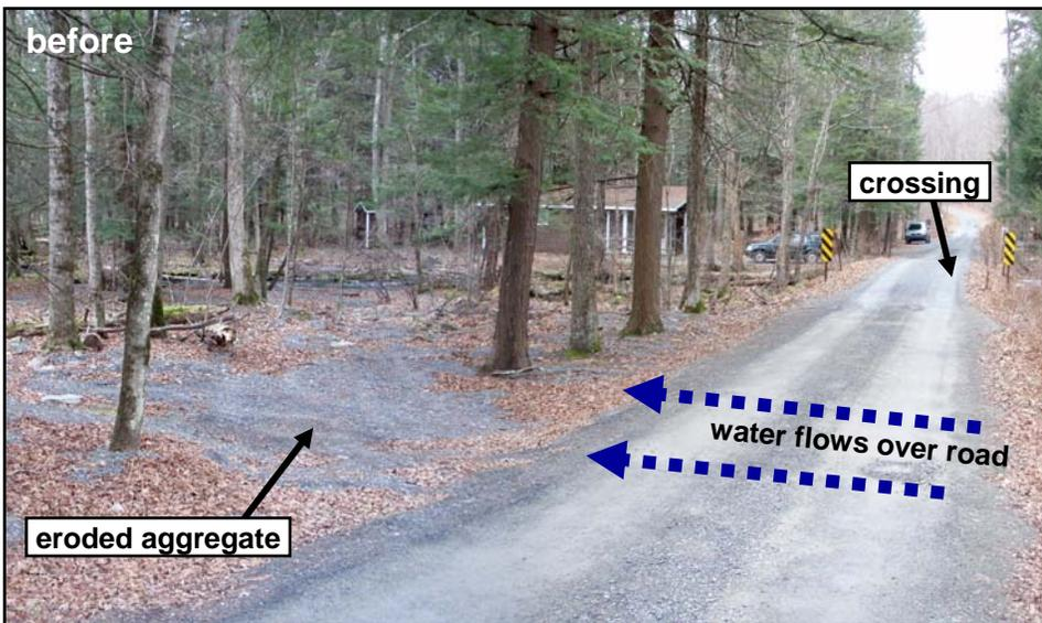
Photo 1. When the undersized stream pipes reach capacity, water flows over the road at this point. Large quantities of aggregate are routinely washed into the floodplain and stream.
