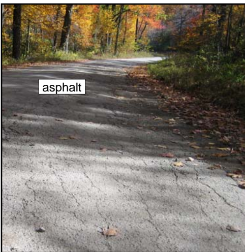
The existing "tar and chip" road is failing. This section of road will be converted to gravel.
