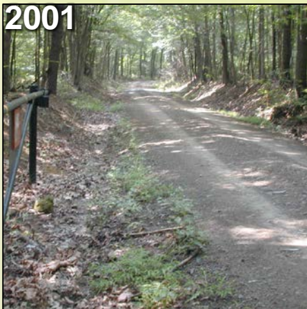
This 15-year-old project in Huntingdon County illustrates the long-term road improvement practices implemented by the program, in this case filling the road profile, adding shallow crosspipes, and driving surface aggregate.
