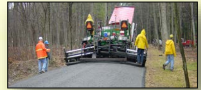
Paver-placement of DSA
