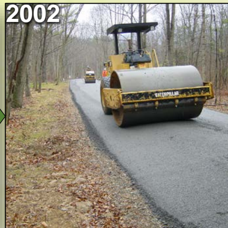
This 15-year-old project in Huntingdon County illustrates the long-term road improvement practices implemented by the program, in this case filling the road profile, adding shallow crosspipes, and driving surface aggregate.
