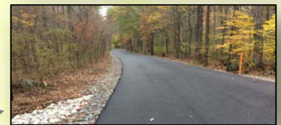
Completed LVR project
