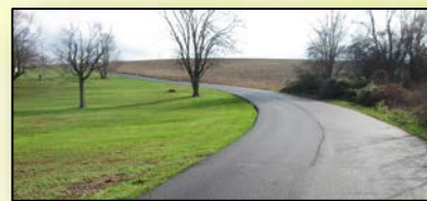
Newly paved LVR
