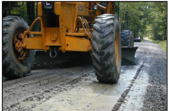
Figure 5. Toothed grader blade used on section 6 to incorporate suppressant into road.
