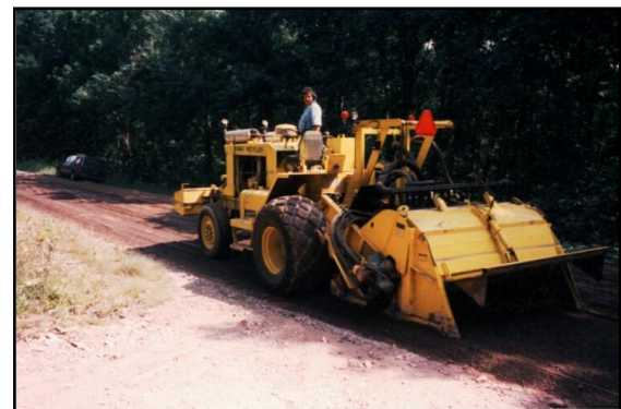
Figure 6. – Bomag Road reclaimer used on section 7 to incorporate suppressant into road.
