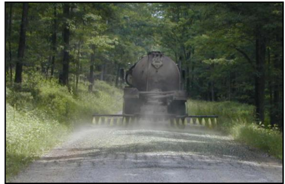
Figure 4. Spray application of topical dust suppressants.
