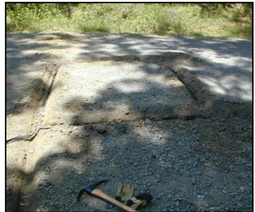
Figure 12. Installation of a buried wire traffic counter.
