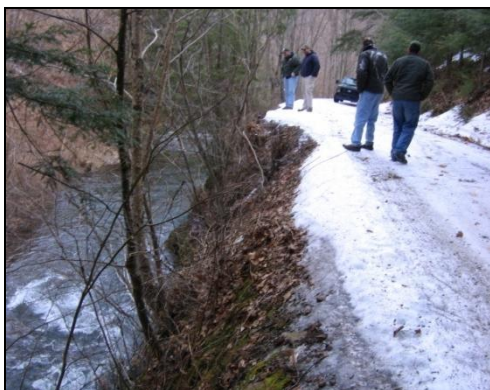
Francis Road (before): The bank instability here was caused by the proximity to the stream.
