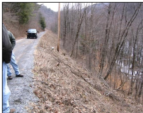
Slate Run Road (before): The bank instability here is caused by the many springs and seeps that saturate the site every year.
