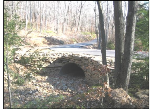
A bottomless arch pipe installed in the Tiadaghton State Forest in 2009.
