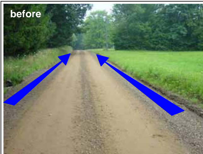
Before: The entrenched road trapped drainage, concentrating it and increasing its erosive potential. After: The elevation of the road is raised, eliminating the right side road ditch and allowing water to sheet flow off the road.
