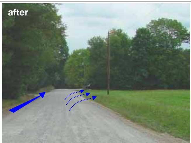
Before: The entrenched road trapped drainage, concentrating it and increasing its erosive potential. After: The elevation of the road is raised, eliminating the right side road ditch and allowing water to sheet flow off the road.
