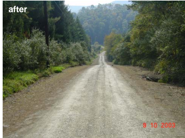
Before and After Shale Placement. Before, severely entrenched road slopes steeply to stream at the bottom of the hill. After, cross-pipes are added to divide drainage and reduce concentrated flow and the road elevation is raised 2' to cover the new pipes.
