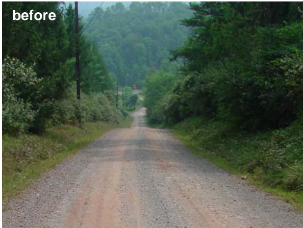
Before and After Shale Placement. Before, severely entrenched road slopes steeply to stream at the bottom of the hill. After, cross-pipes are added to divide drainage and reduce concentrated flow and the road elevation is raised 2' to cover the new pipes.
