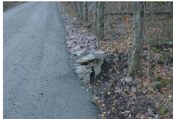
Figure 2. AFTER Filling: Shallow crosspipe installation with minimal disturbance.
