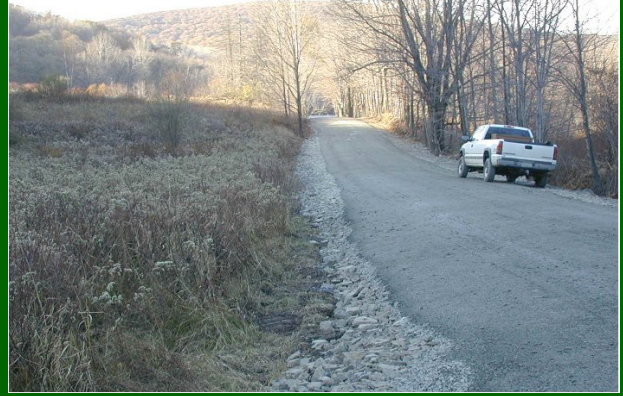
Figure 4. AFTER filling: Filling the road achieves proper drainage without collecting water.
