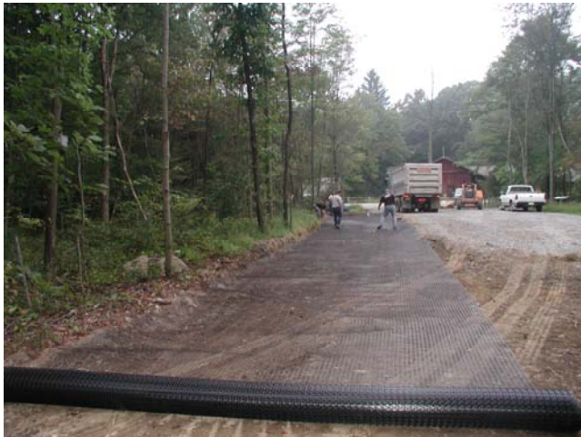
Above: Construction of the bus parking lane. Geogrid® was used to add support and tensile strength.
