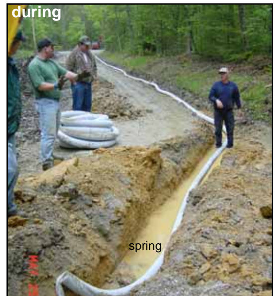
Photo 2. Pre-fabricated underdrain was used to collect subsurface water from under the road and both ditches.
