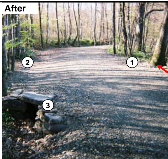
Photo 1 & 2. This Before & After sequence illustrates many of the techniques used on the site. Before, road drainage continued in the ditch for almost 2000' where it emptied into a stream. After, this section does not affect the stream.
