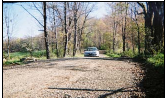
Photo 5: New Crosspipe installation with gradebreak. Top of gradebreak obscures car in bottom of gradebreak.
