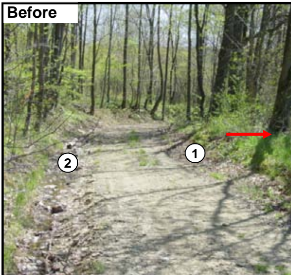
Photo 1 & 2. This Before & After sequence illustrates many of the techniques used on the site. Before, road drainage continued in the ditch for almost 2000' where it emptied into a stream. After, this section does not affect the stream.
