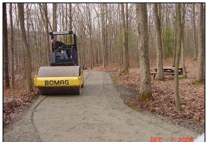
Photo 5. Compaction of paver-placed Driving Surface Aggregate
