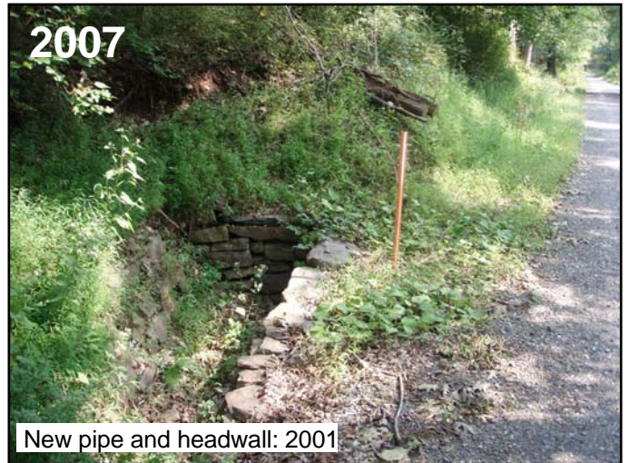
Photo 2 & 3. Six years after construction, the new pipe and headwall on the right is still stable. The existing pipe on the left was left alone. The unstable bank around the pipe inlet is a constant source of sediment and could clog the pipe if part of the bank were to collapse.
