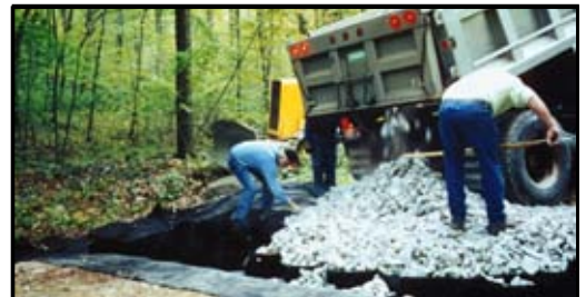
Photo 5. Geocell and stone fill for water crossing.
