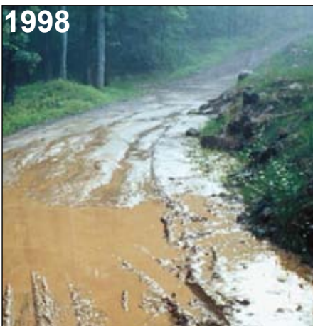
Photo 1 & 2 This low lying section of road was frequently flooded. By addressing surface drainage and reinforcing the overflow area, road impacts were minimized.
