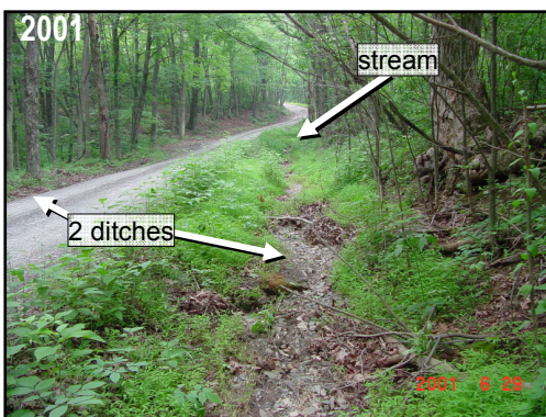
BEFORE. Entrenched road traps runoff in ditch, transporting it to stream. Heavy canopy and insufficient cover to install crosspipes.
