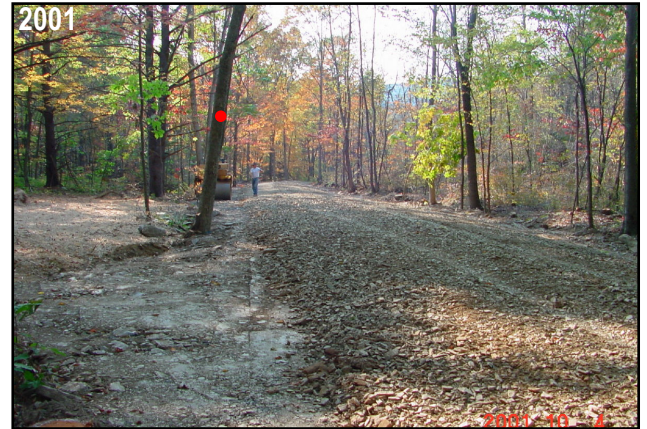
DURING. Entrenched road is filled with shale. Trees are selectively thinned.
