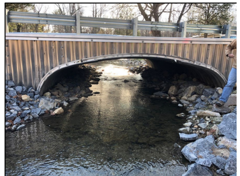
19' w x 6' h structure showing low flow channel and bank margins (Northampton)
