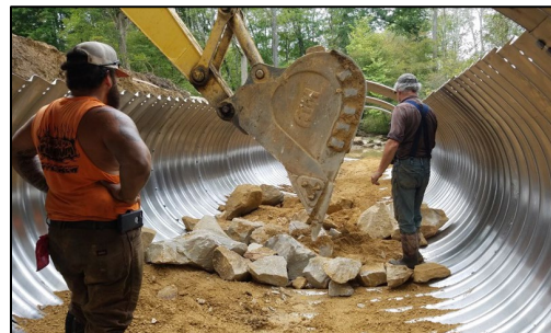
Photo 2: Placing large material during pipe assembly.
