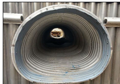
Pipe arch or "squash pipe" (6' wide) (CDGRS)
