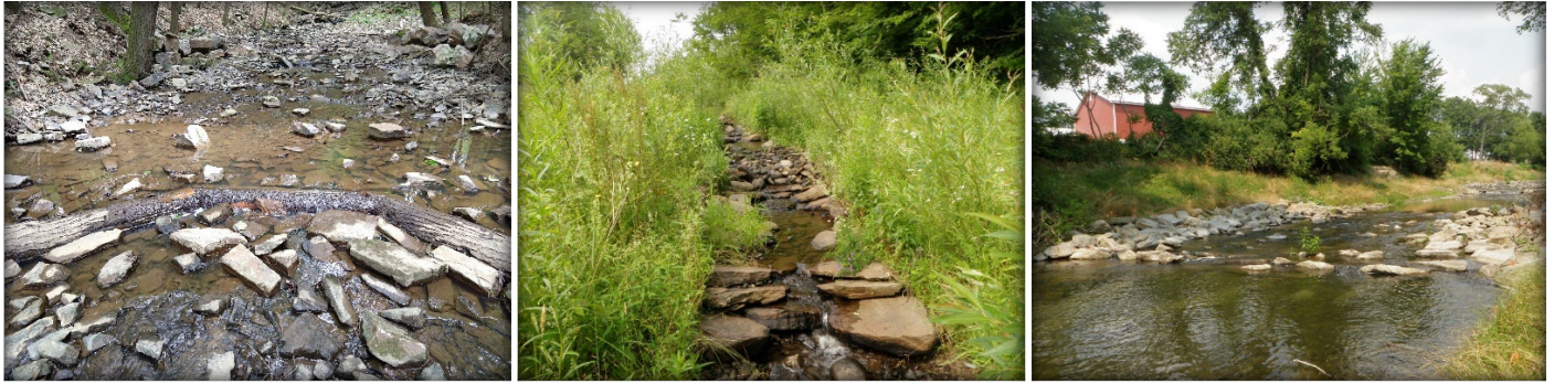
Figure 1: From left to right, log cross vane with throat log; rock clusters and cascade; and constructed riffle.
