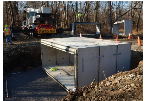
Assembly of a 16’w x 6’ h concrete box culvert (Montgomery).
