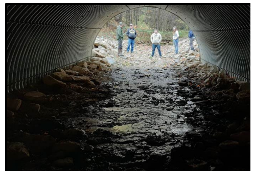
Completed 16' w x 10' h pipe arch (Crawford).
