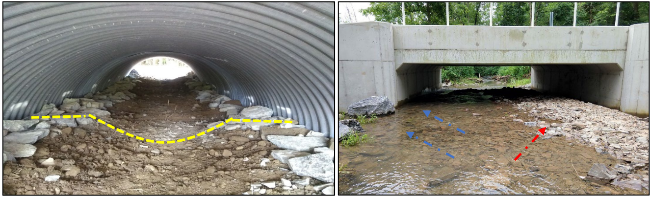
Figure 3: The photo on the left shows a properly constructed streambed with a low flow and bankfull channel, along with bank margins. The photo on the right shows a structure that did not have a properly constructed channel, and the resulting sediment deposition at the inlet is forcing the flow to the side of the structure.
