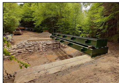
Spread footer bridge installation (Indiana)
