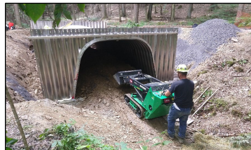
Photo 2: Placing fine material in a 8'w x 6'h bottomless arch with a walk-behind skid steer.
