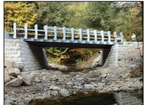
Completed 32' span GRS-IBS bridge (Tioga).
