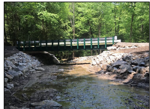
Completed 50' span (~25' channel) spread footer bridge (Indiana).
