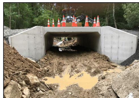
Bottomless concrete box culvert (Cumberland)
