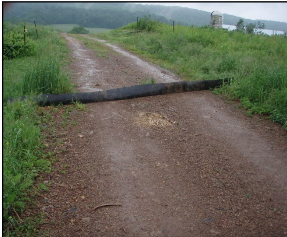
Completed Conveyor Belt Diversion
