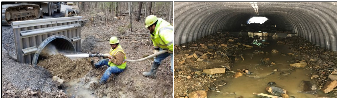
Figure 6: The photo on the left shows washing of fine material into a 6'w x 4'h pipe arch (squash pipe) using a fire truck. The photo on the right shows the washing process between tanker loads and view of a baffle grade control.
