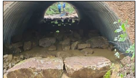
Photo 4: Large material placed in a 12'w x 6'h arch pipe before placing streambed.
