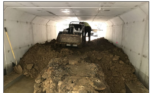
Photo 3: Placing fine material inside a bottomless concrete culvert with walk behind skid steer.
