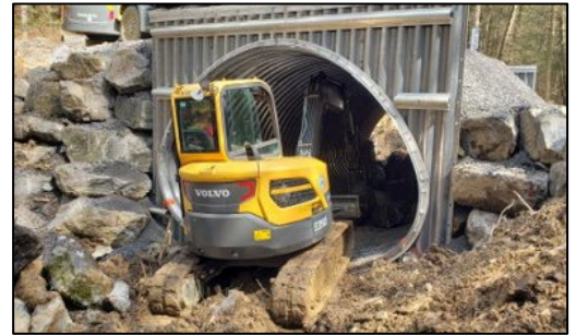
Photo 1: Placing larger material in a 15'w x 10'h pipe arch (squash pipe).
