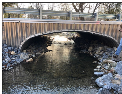
19' w x 6' h structure showing low flow channel and bank margins (Northampton)
