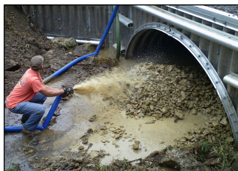
Washing fines into the streambed on a 12' w x 4' h pipe arch (Jefferson).
