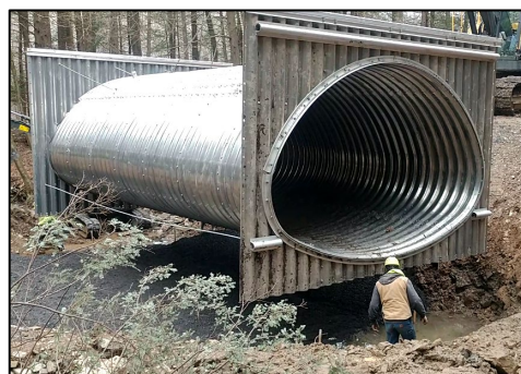
Installation of a 15' w x 10' h pipe arch that was assembled on site (CDGRS).
