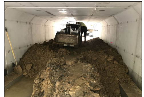
Walk-behind equipment being used to place streambed in 12' w x 6.5' h bottomless concrete box (Cumberland).
