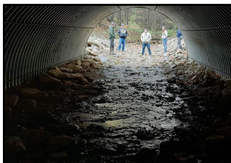
Completed 16' w x 10' h pipe arch (Crawford).
