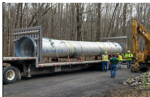
Delivery of a fully assembled 6' w x 4' h x 40' l pipe arch (CDGRS).
