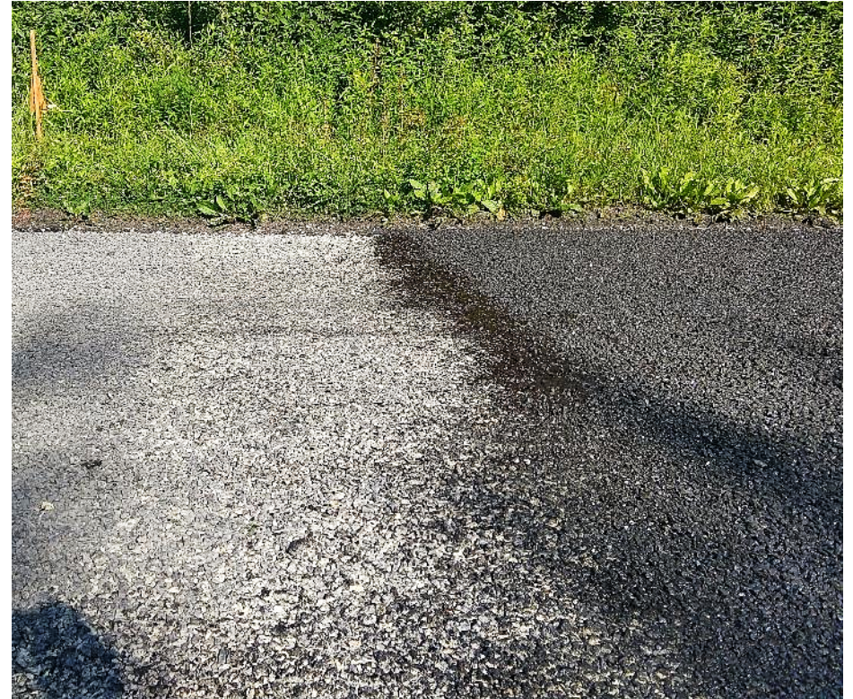
#67 base left with #8 topcoat right
