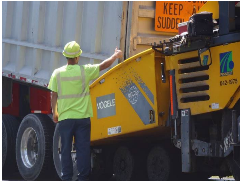
Delivery of asphalt mix to paver
