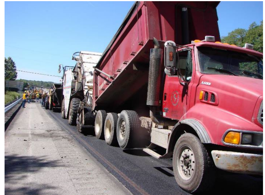
Delivery of asphalt mix to materials transfer vehicle
