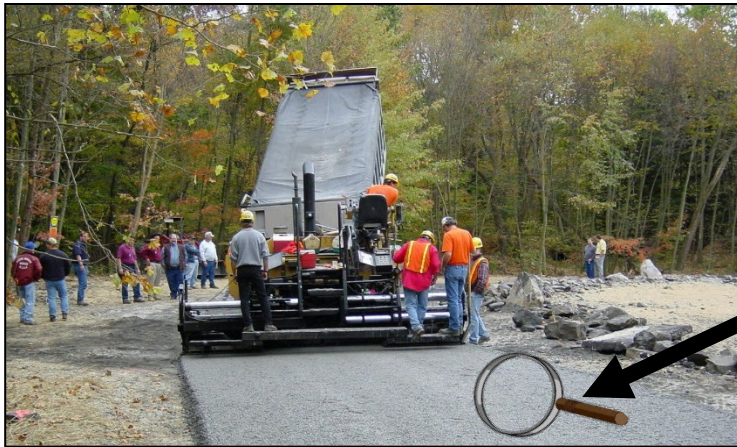
Figure 1 - Placement of DSA through a paver
