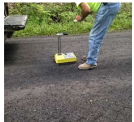
Figure 4: Compaction Testing with Nuclear Density Gauge
