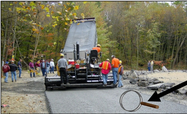
Figure 1: Placement of DSA through a paver.
